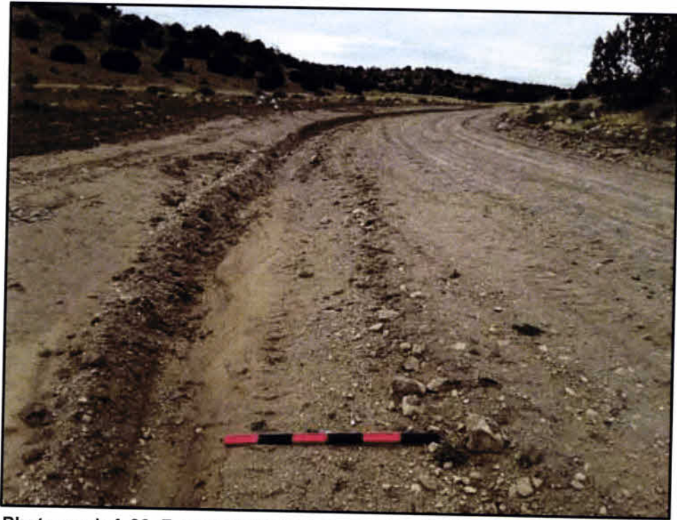
Photograph A.83. Feature 30, DP-42; roadside ditch/water bar, view upgradient.
