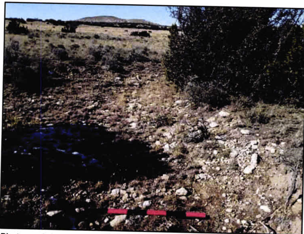
Photograph A.68. Feature 24, DP-33; swale/erosional feature, view downgradient.
