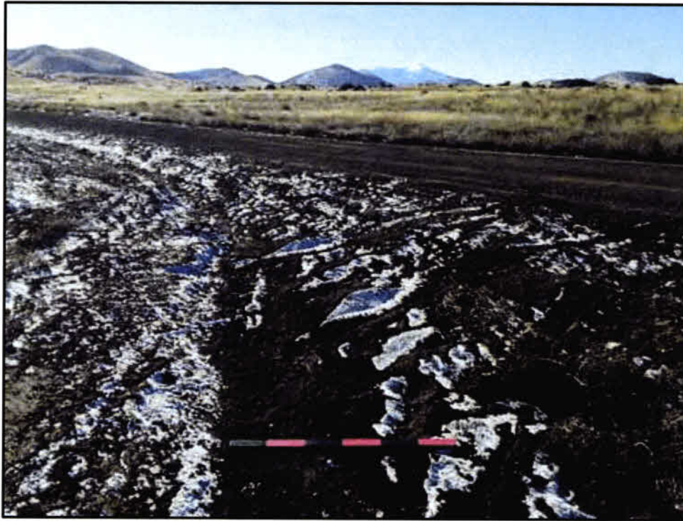
Photograph A.23. Feature 9, DP-11; human-made road water bar, view upstream.
