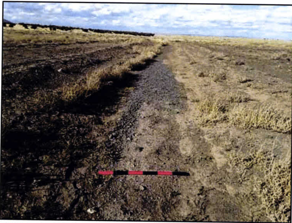
Photograph A.32. Feature 13, DP-15; human-made road water bar, view downstream.
