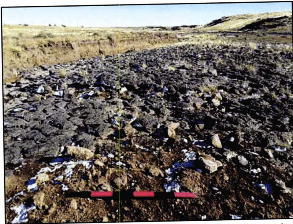
Photograph A.30. Feature 12, DP-14; sheet flow concentrating into a rocky swale, view downgradient.
