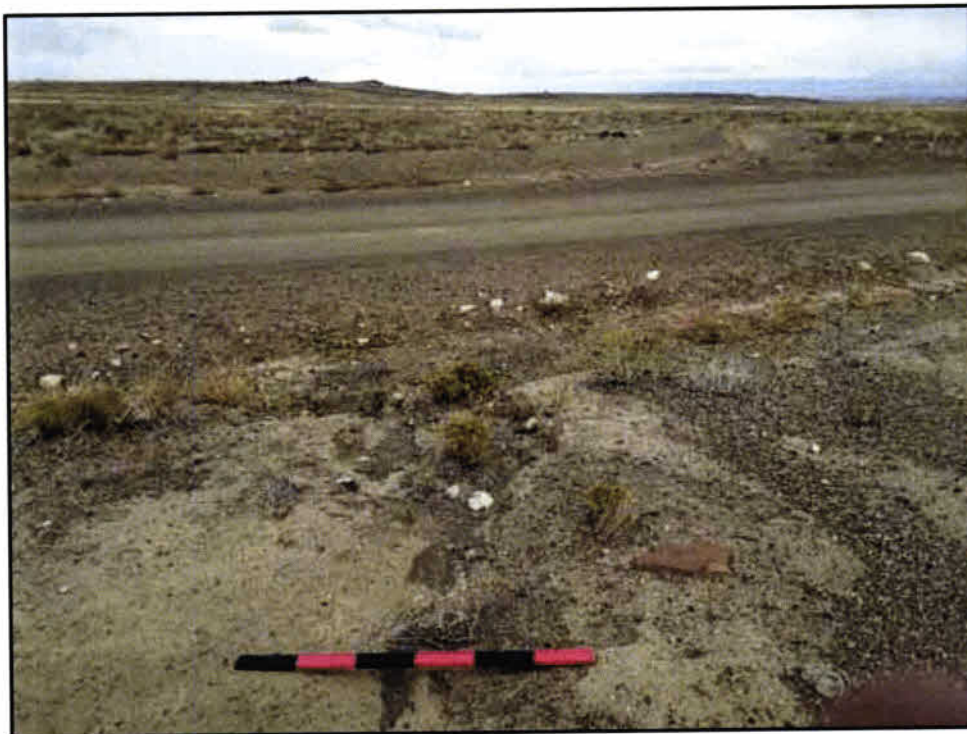
Photograph A.10. Feature 4, DP-52; human-made road water bar, view downstream.
