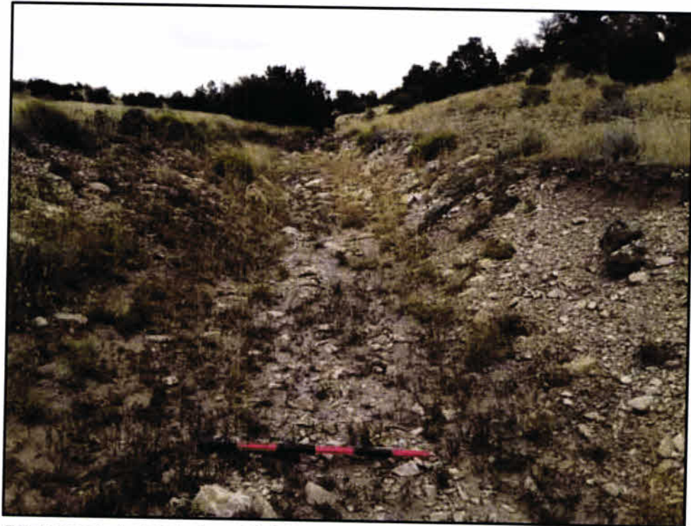
Photograph A.87. Feature 31, DP-43; erosional feature, view upgradient.
