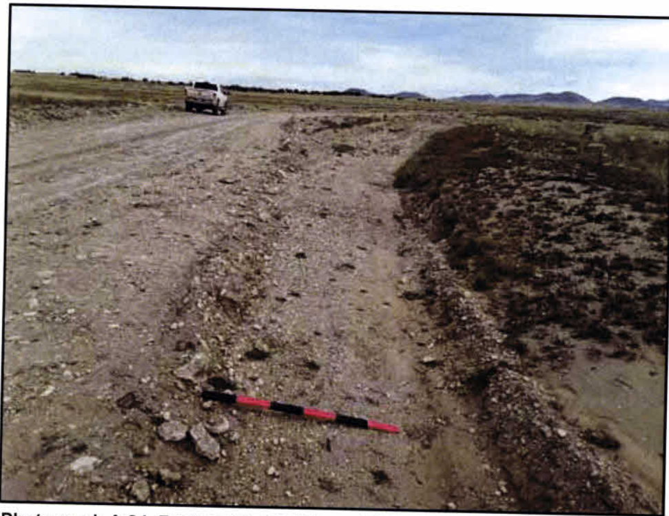
Photograph A.84. Feature 30, DP-42; roadside ditch/water bar, view downgradient.
