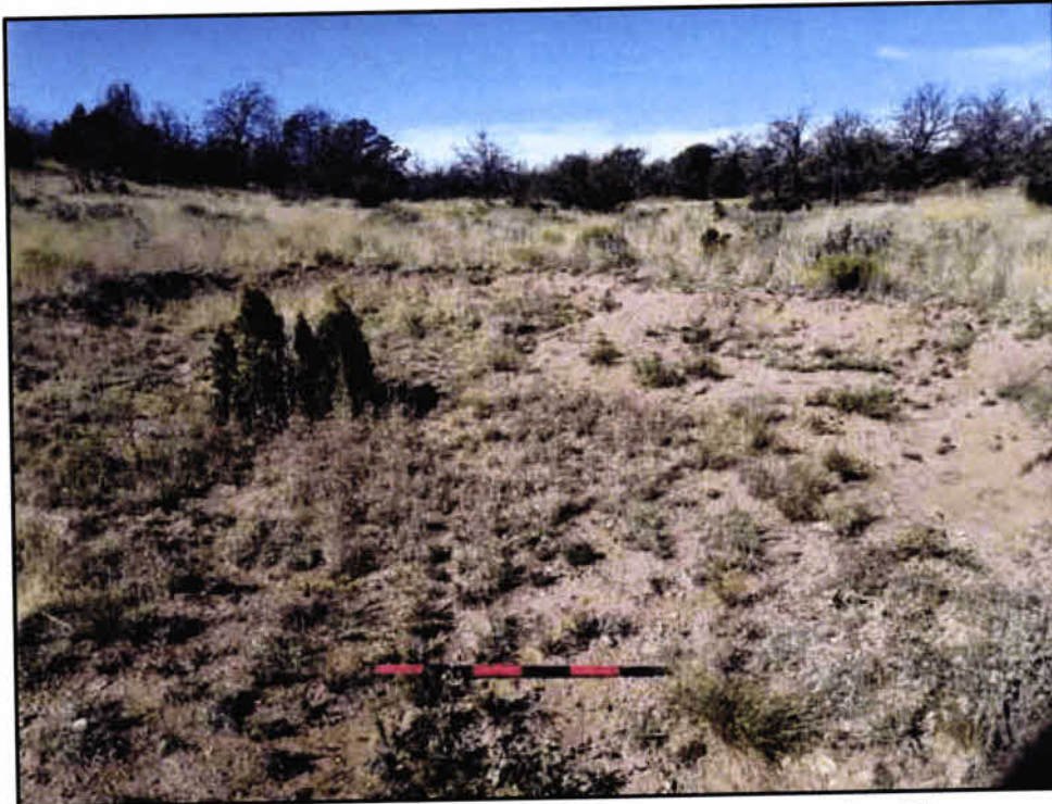
Photograph A.133. Feature 45, DP-65; erosional feature/swale with headcutting, view upgradient.
