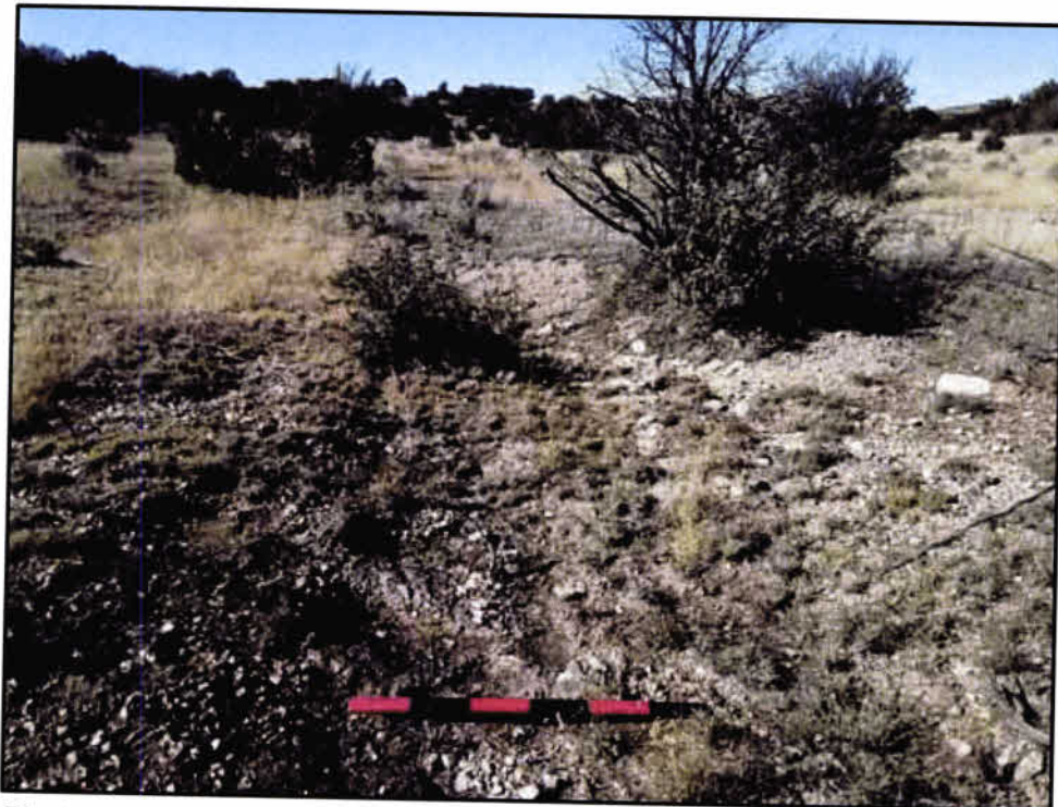
Photograph A.72. Feature 25, DP-40; erosional feature, view downgradient.
