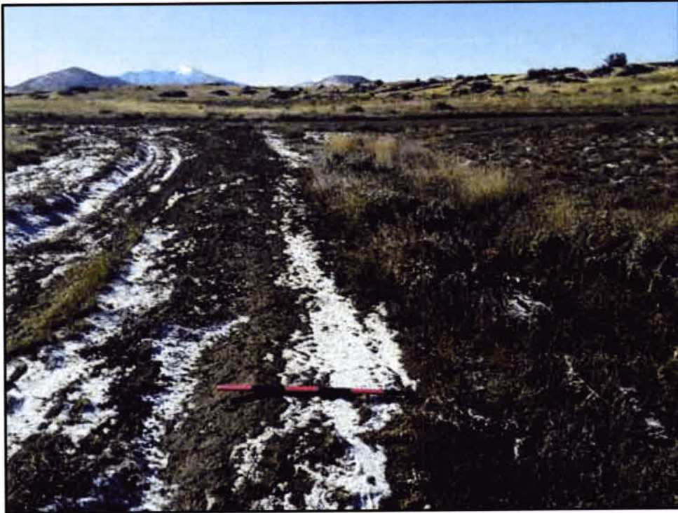
Photograph A.25. Feature 10, DP-12; human-made road water bar, view upstream.
