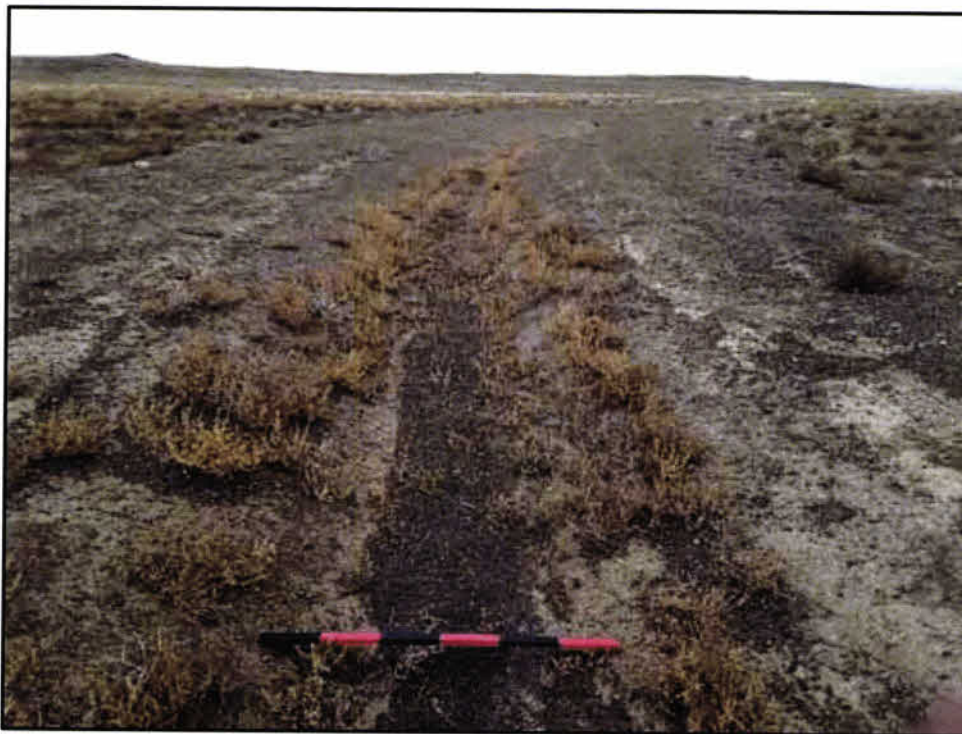
Photograph A.8. Feature 4, DP-4; human-made road water bar, view downstream.
