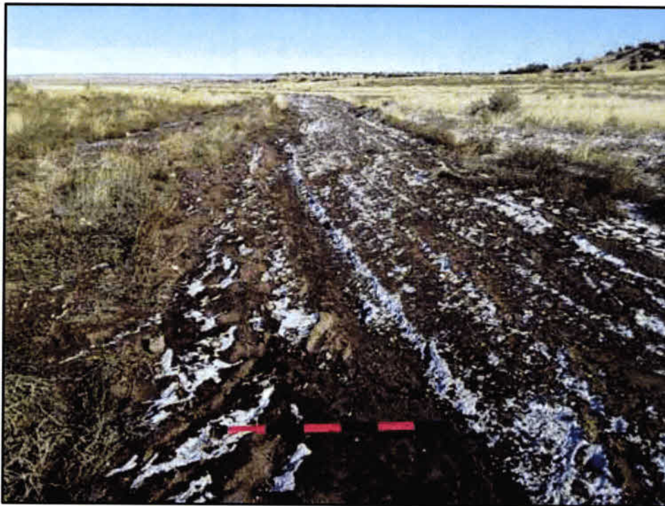
Photograph A.24. Feature 9, DP-11; human-made road water bar, view downstream.
