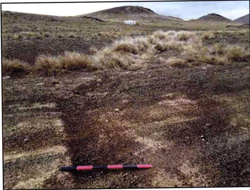
Photograph A.13. Feature 6, DP-6; human-made road water bar/swale, view upstream.
