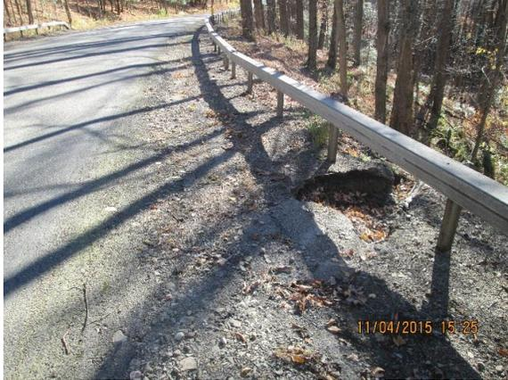
DETERIORATED AND WASHED OUT WEST SHOULDER
