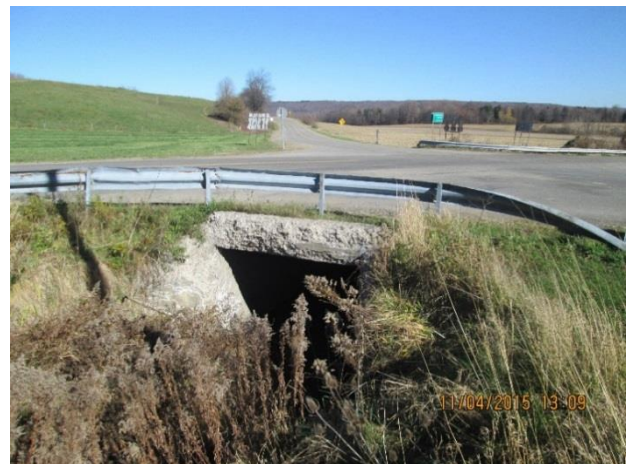
CULVERT AT INTERSECTION OF BARD RD AND CR 85 LOOKING NORTH
