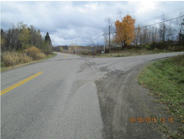
INTERSECTION OF HALL RD AND BARD RD (CR 72) LOOKING EAST
