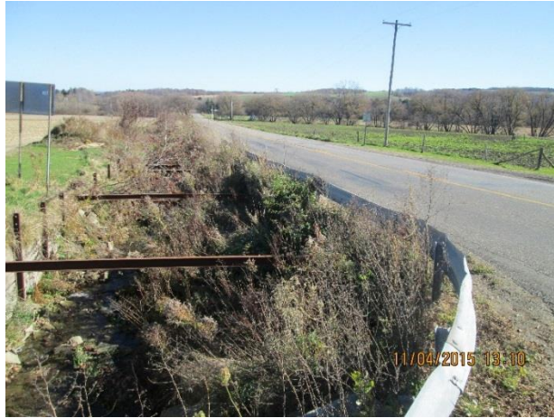
INTERSECTION OF BARD RD AND CR 85 NORTHEAST CORNER LOOKING EAST
