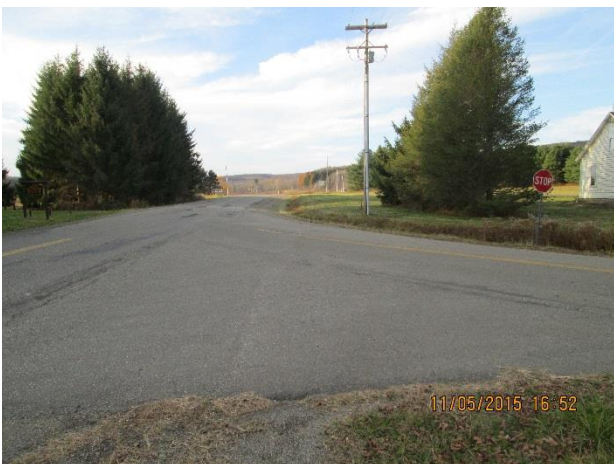
NORTHERN INTERSECTION OF ERWIN RD (CR 85) AND CR 66 LOOKING NORTHWEST
