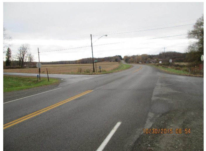
INTERSECTION OF BARD RD AND SHUMLA RD LOOKING NORTHEAST
