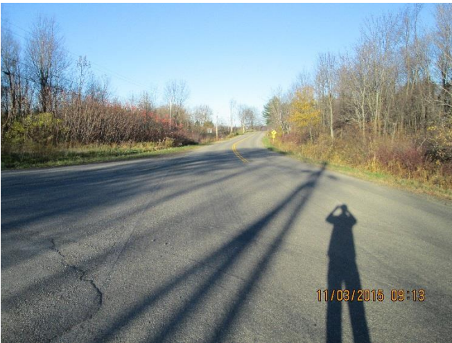
INTERSECTION OF BARD RD AND HALL RD LOOKING WEST
