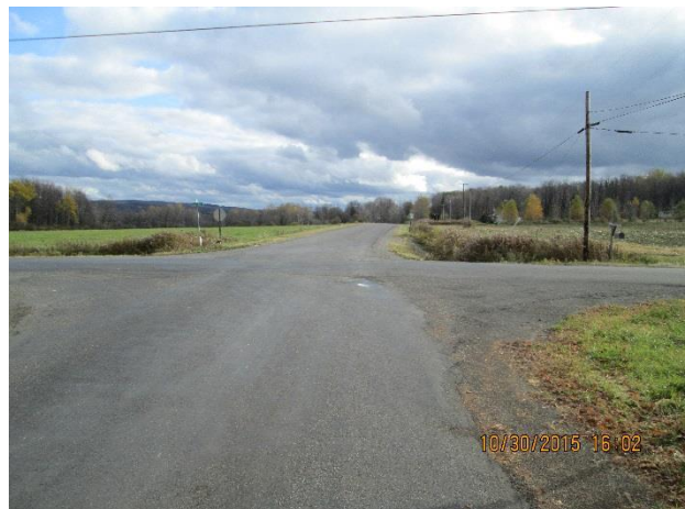
INTERSECTION OF HALL RD AND HOOKER RD LOOKING SOUTH
