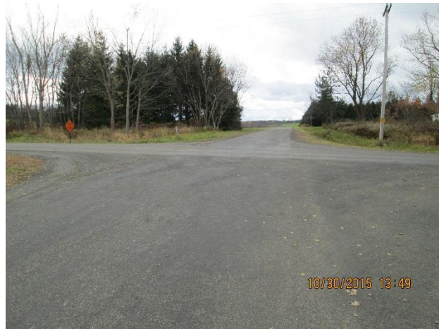
INTERSECTION OF HALL RD AND CASSADAGA RD LOOKING SOUTH
