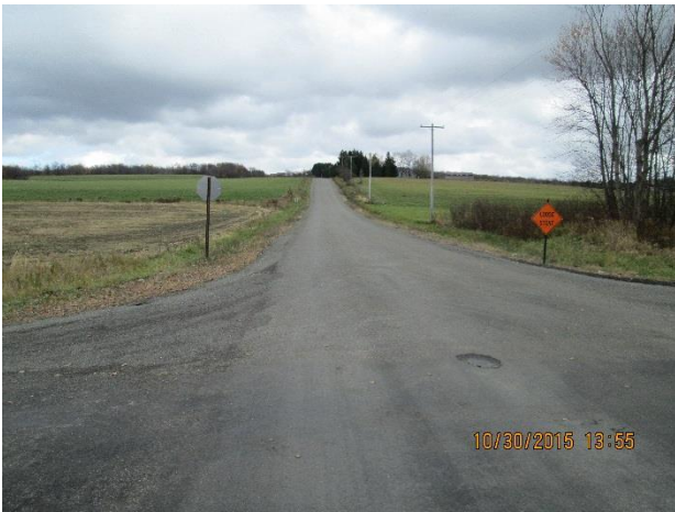
INTERSECTION OF CASSADAGA RD AND HALL RD LOOKING EAST
