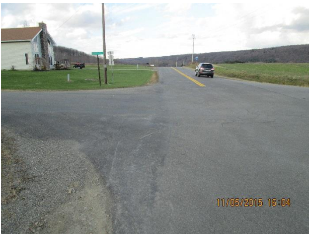
INTERSECTION OF BOUTWELL HILL RD AND CR85 LOOKING NORTH
