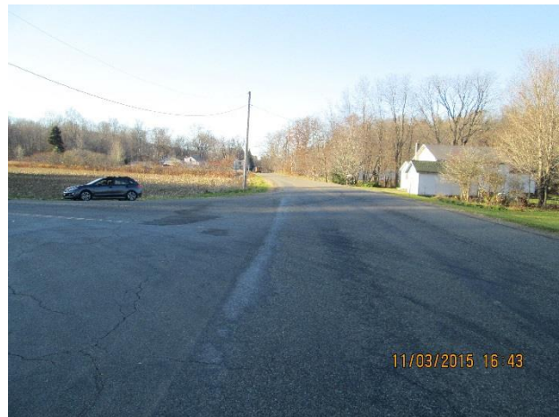
INTERSECTION OF CR 66 AND BATES RD (CR 64) LOOKING NORTHWEST
