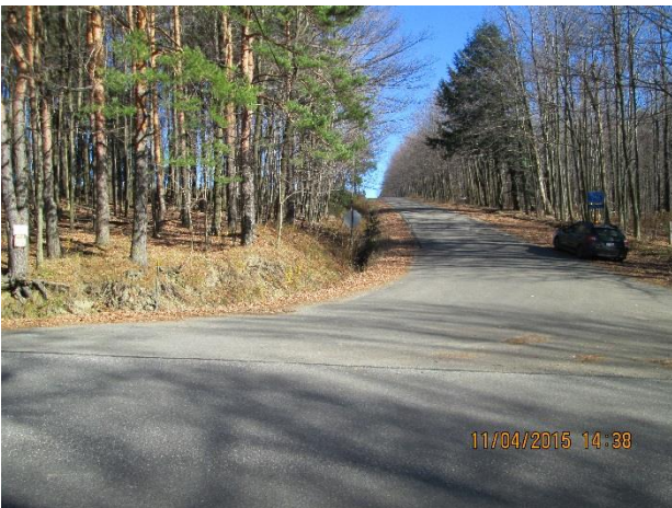
INTERSECTION OF WEAVER HILL RD AND PLANK RD
