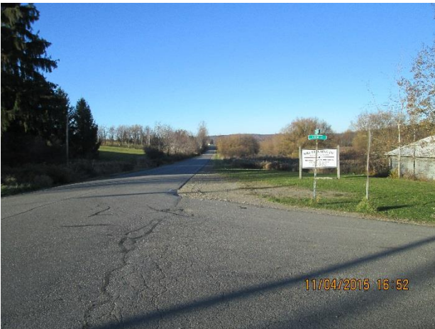
INTERSECTION OF COOK RD AND ROOD RD (CR 77) LOOKING NORTH
